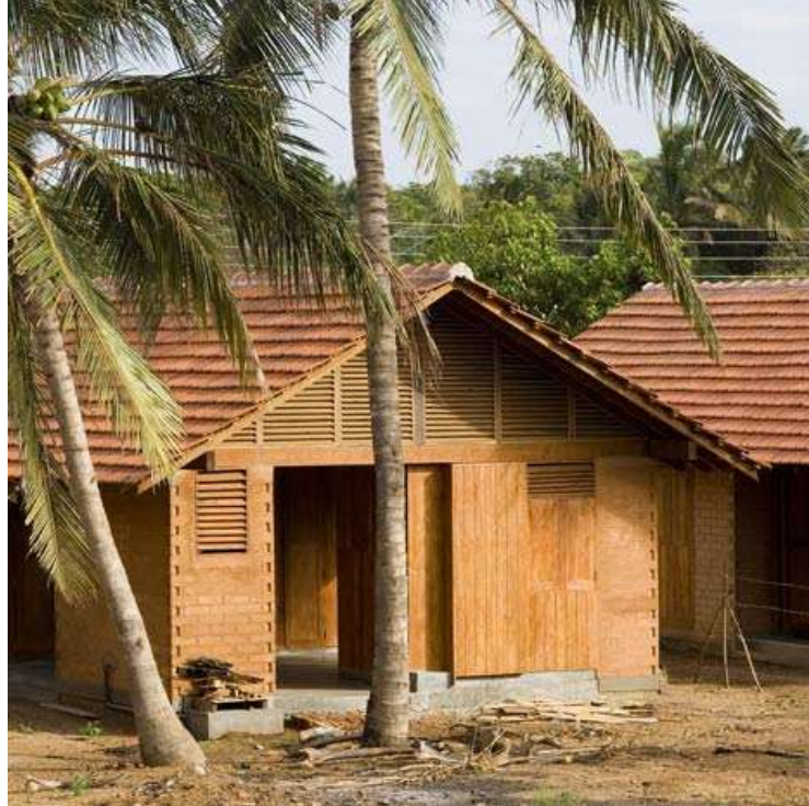
Figure 2 Climate-responsive post-tsunami housing in Sri Lanka using vernacular design principles, local materials, natural ventilation, and traditional roofing systems. Source: Author's previous publication (Ewiss & Hajismail, 2026), with original reference from Dezeen (2013).
